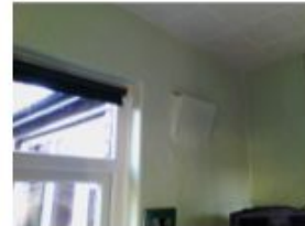
Figure D: Showing cool area and draught from uncontrolled vent in ground floor kitchen.
