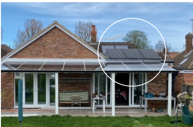
Example of a solar panel array on the roof of a covered verandah at the rear of the property.
