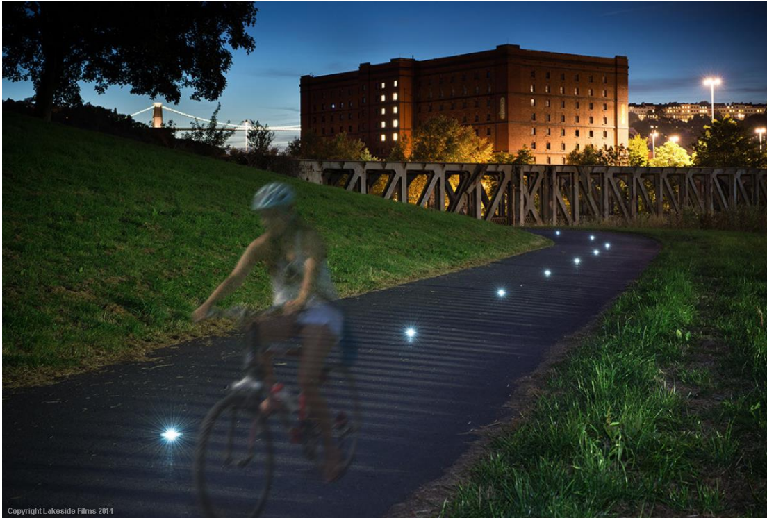
Figure 5.3: Example of low-level LED lighting of cycle paths
