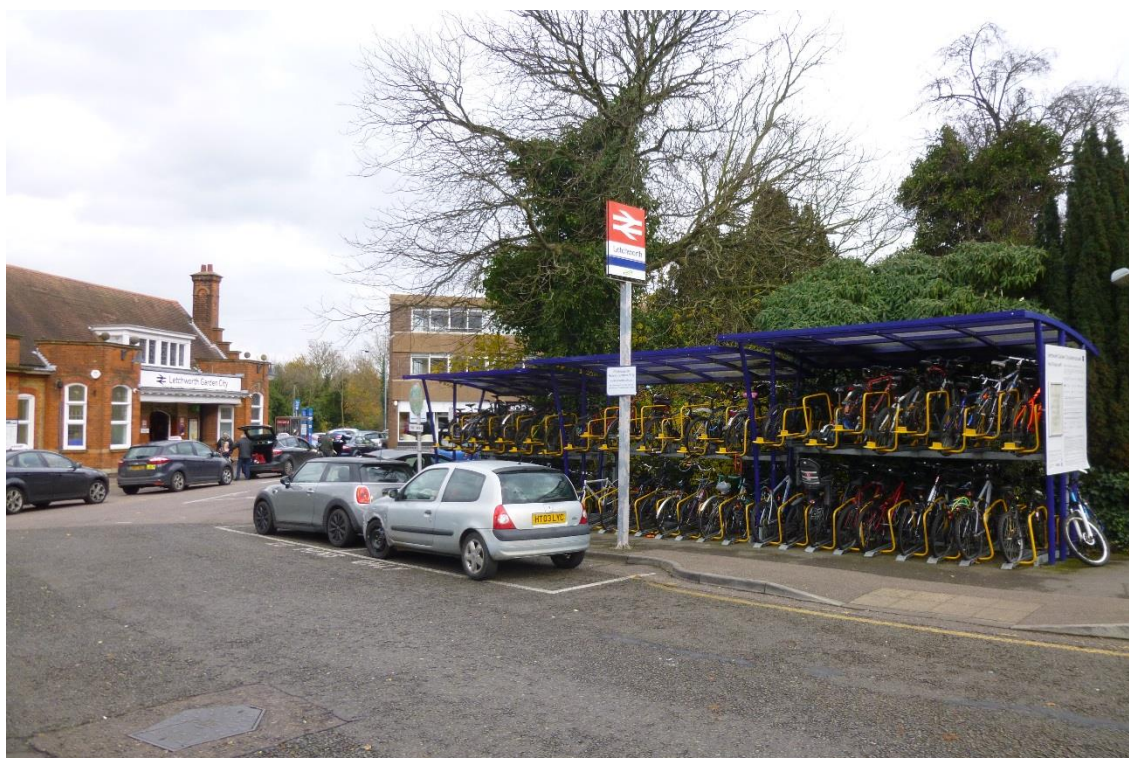
Figure 2.10: Cycle parking at Letchworth train station
