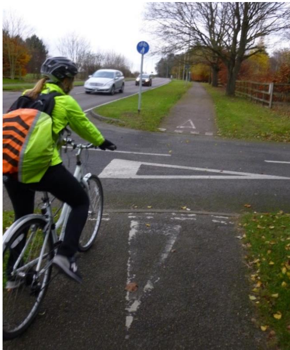
Figure 5.15: Side road has priority over cycle track between Hitchin and Letchworth
