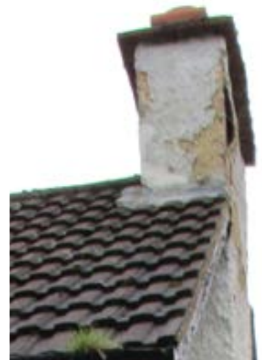
Blown render and blocked gutter
