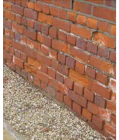
Damaged brickwork and mortar
