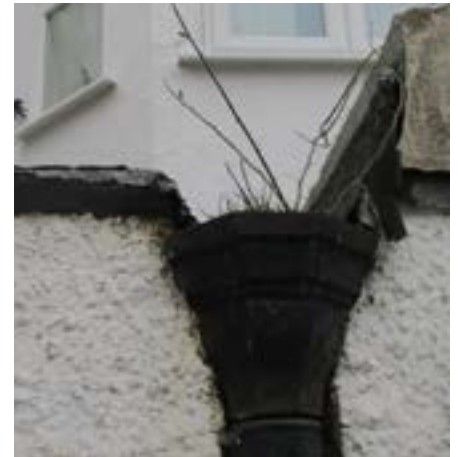
Blocked hopper head
