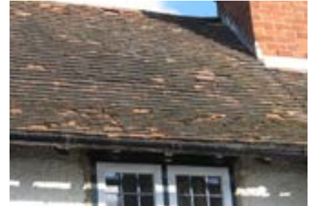
Slipped roof tiles
