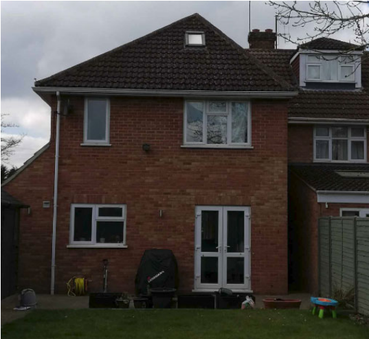
Image shows current maintenance gap between properties
