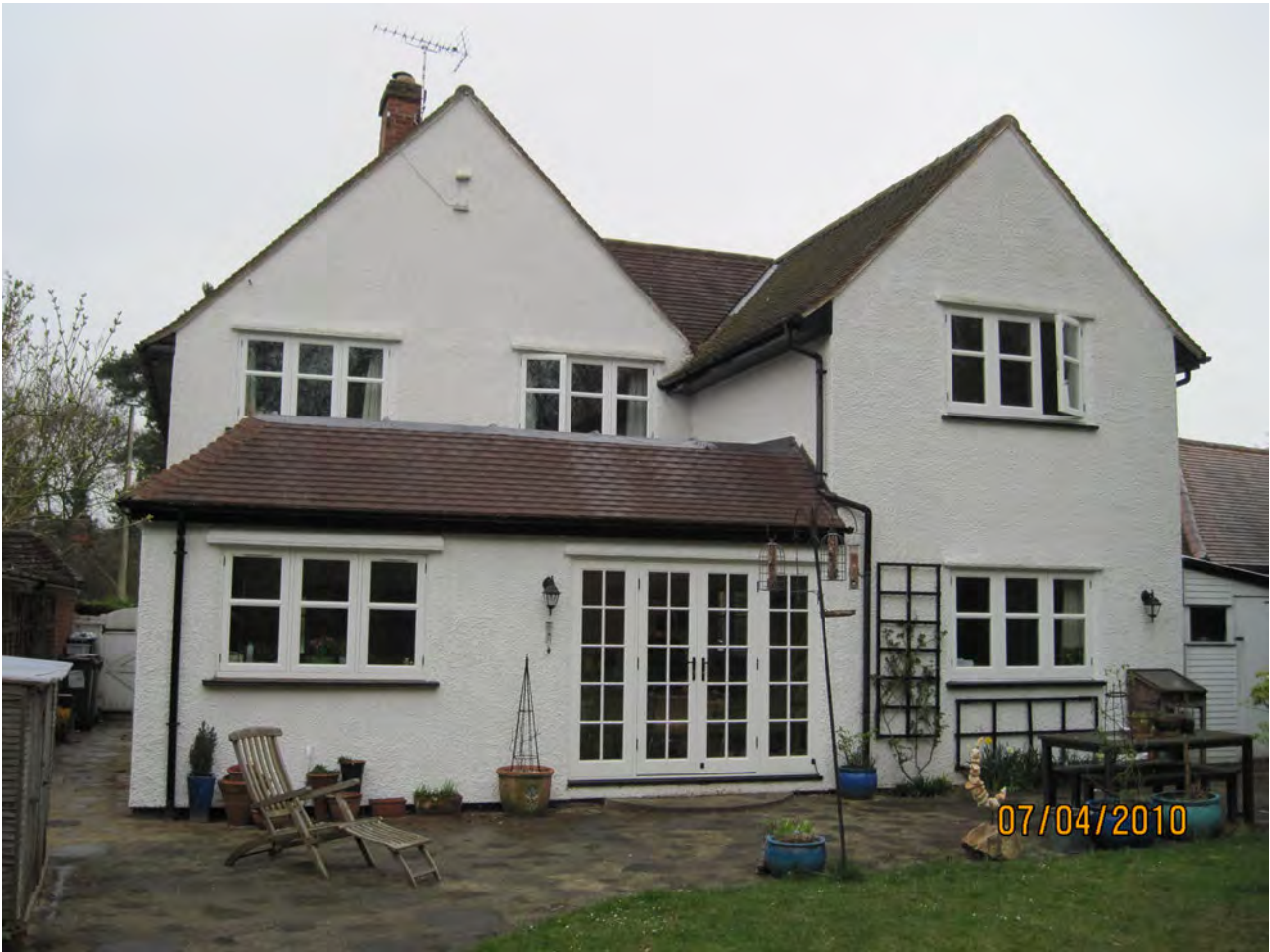
Rear of house without rooflights which were consent in 2021
