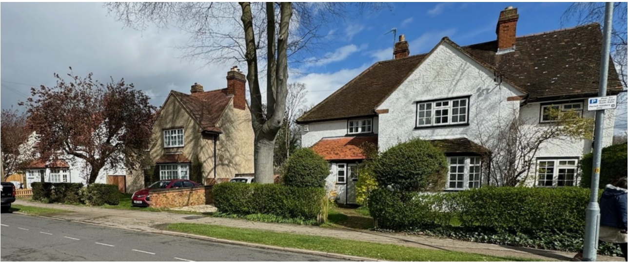
26, 28 and 30 South View
